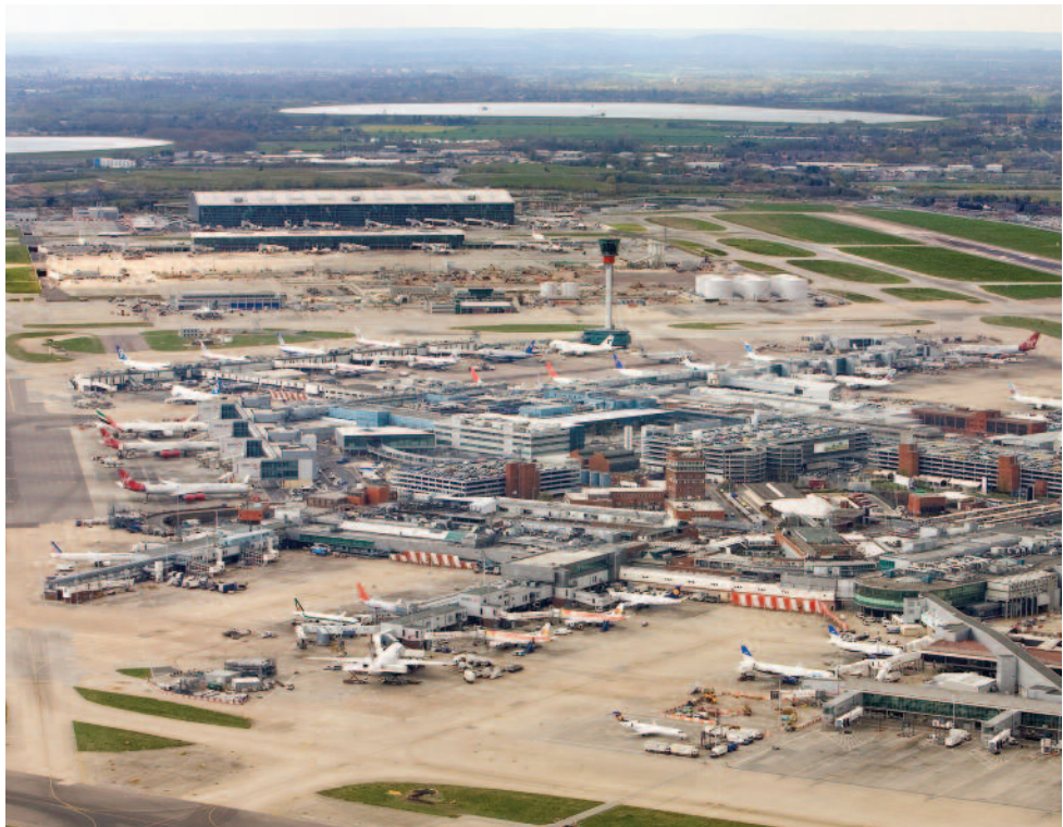
Figure 18 Aircraft on the ground at Heathrow Airport. Until the 11 December 2005 incident, Heathrow drew about half of its 21 million litres daily consumption of aviation fuel from Buncefield via the West London Pipeline System
