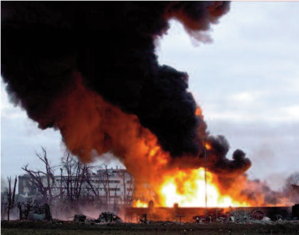
Figure 19 The remains of the fire in Tank 12 at Buncefield, on the BPA depot. This was the largest tank on the Buncefield site and could store 19 million litres of aviation fuel
