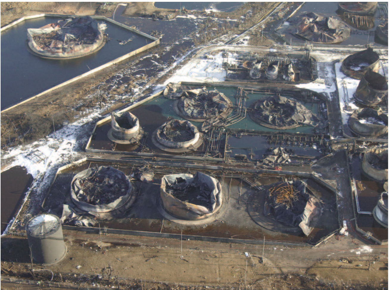
Figure 1 View from the west of the Buncefield Hertfordshire Oil Storage depot after the fires were all out. Tank 912, from which the petrol feeding the vapour that exploded escaped, is in the centre of the bund at the bottom of the picture. Cherry Tree Lane, a public road, cuts diagonally across the upper part of the picture and is flooded ('Lake Buncefield'). Across the road are the remains of Tank 12, a large aviation fuel storage tank. The roof of the fire pump house can be seen embedded in foam at middle left. The adjacent fire water lagoon is covered in escaped fuel
