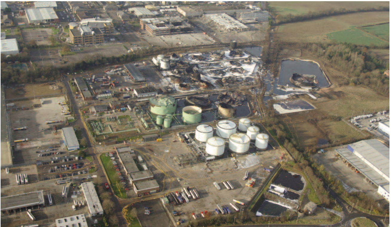
Figure 13 The Buncefield site and surrounding ground at the time the police handed the investigation to the COMAH Competent Authority
