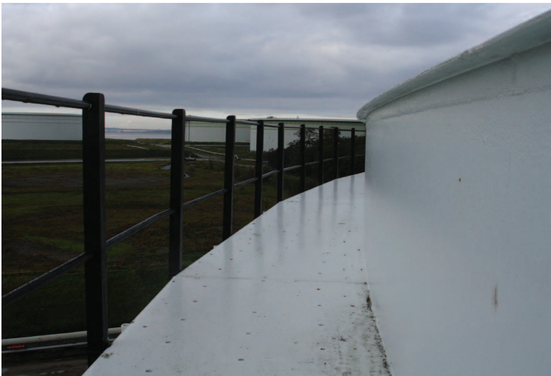
Figure 15 Top girder (walkway) on floating roof tank
