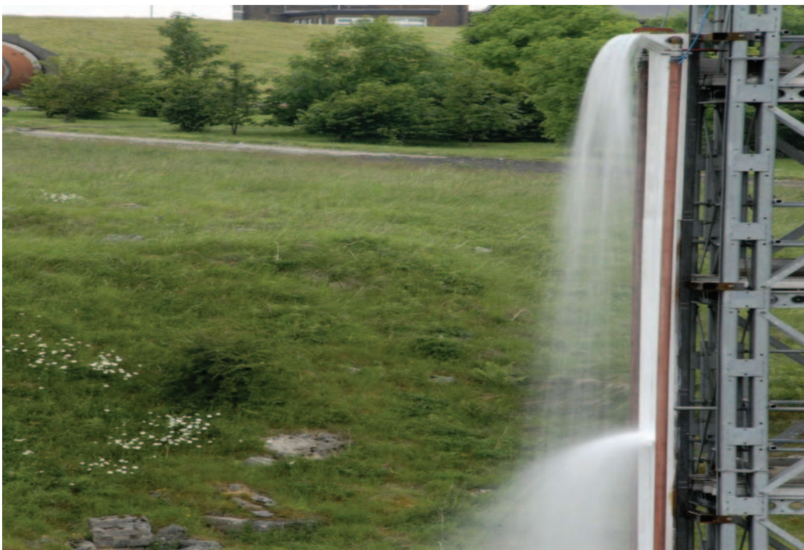
Figure 14 Intersection of free cascades from a Type A tank with a deflector plate
